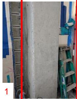
Photos of Completed FRP Installation Process
