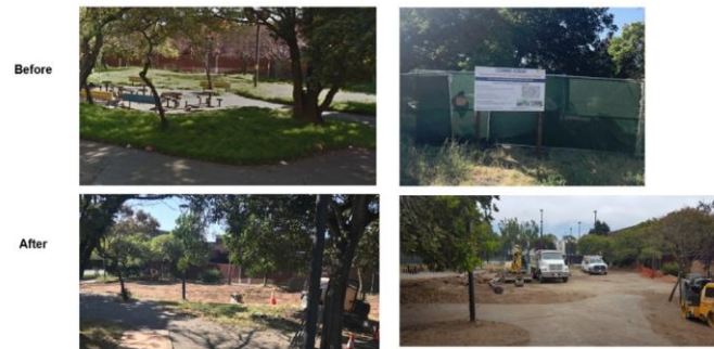
Site Prep for temporary clinic at Ella Hill Hutch Community Center
